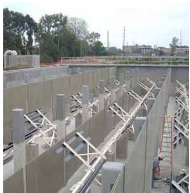
Sludge Flights were supplied for this large municipal project.
