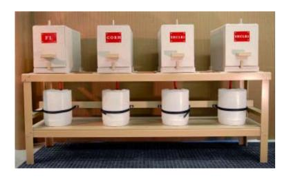
Splash cabinets for refilling chemicals with quick-connect hoses from tank trucks.
