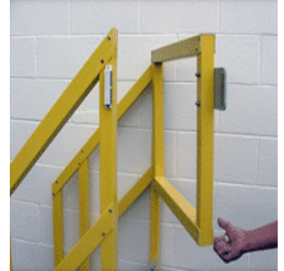
Custom designed swing gate, self-closing using stainless steel hinge and magnetic latch.
