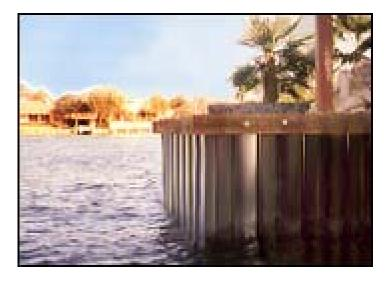
SuperLoc<sup>™</sup> Composite Sheet Pile System, a fiber reinforced polymer (FRP) composite system, is manufactured by the pultrusion process and is designed and manufactured to provide a solution for deteriorated waterfront structures subjected to the harsh marine operating environment.
