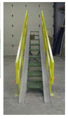
(bottom middle photo) Combination pedestrian stair and hand truck ramp. This unit was fabricated with wide flange beams set on edge to act as runners for hand truck wheels and also to allow workers to use the unit as stairs. Handrail on both sides meets OSHA specification. Ramp/stair unit leads to a raised platform used for mezzanine storage.
