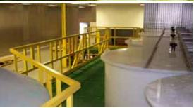
Food processing plants require unique solutions. Preventing worker fatigue on conveyor lines and a clean, safe environment are primary considerations. Ultra's fiberglass platforms, staircases, guardrail and machine access step-ups or walkovers can keep processes moving efficiently and comply with USDA guidelines. Slip resistant grating is used for consistent washed or wet areas to avoid slip hazards. Sealed fiberglass is used to prevent bacteria growth and comply with USDA requirements.
