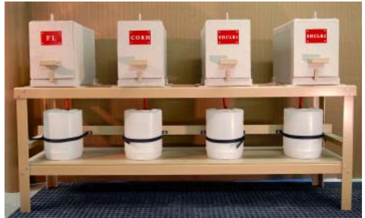
Splash cabinets for refilling chemicals with quick-connect hoses from tank trucks.
