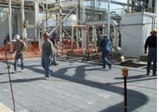
Covers are light in weight, but strong. They can be designed to carry almost any loading from man loads to machinery loads. A variety of decking materials are available. Lightweight structurals save both freight and assembly dollars.
