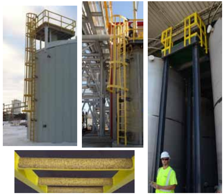
Non-skid UltraGrit™ coated rungs
